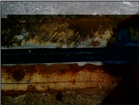
Complete BEJS joint installation.
