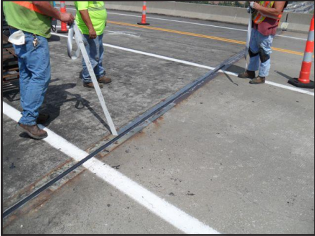
11:00am Removing duct tape from top of metal angles.
