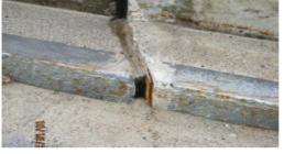
The joint seal splices (left photo) seem to be holding up well. The seal is supplied in 6.56 LF (2 m) lengths and is bonded end to end in the field with a silicone adhesive prior to insertion into the joint. The silicone sealant bead that runs the length of the seal and bonds to the steel is still holding up well for the most part.
