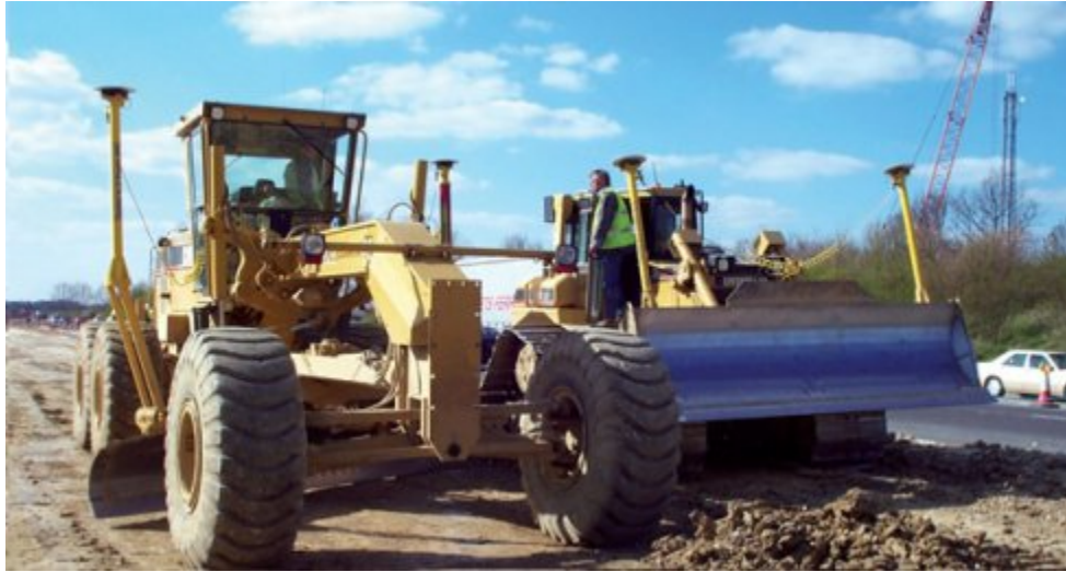
Figure 2.1 – Motor Grader & Dozer outfitted with 3D Machine Control System from Trimble
